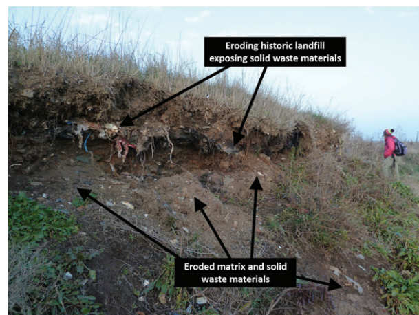
FIGURE 3 | Erosion of solid waste materials from East Tilbury landfill in the Thames Estuary (Source: Dr. J. H. Brand, January 23, 2017).
